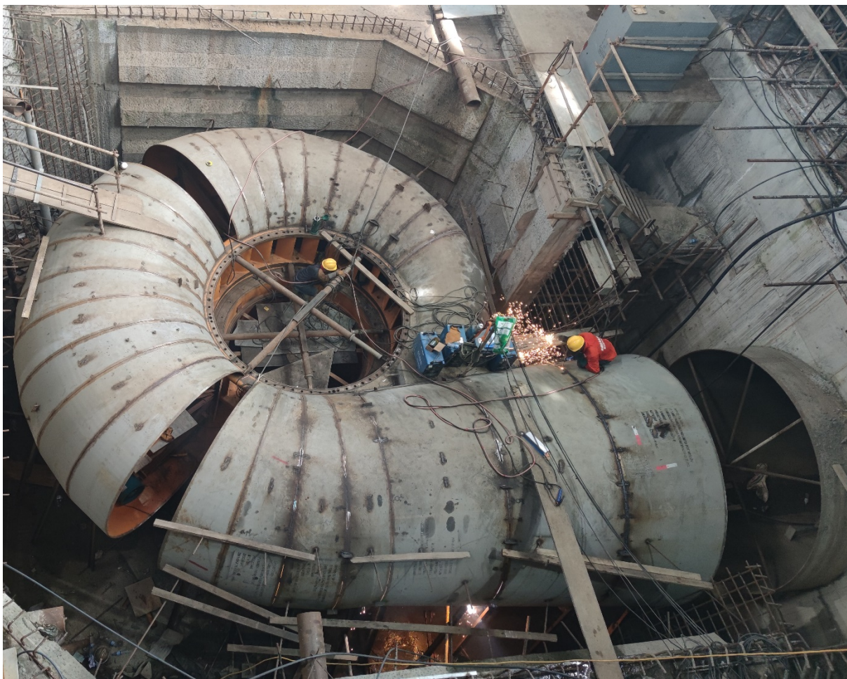
Figure 2 The spiral case of Edevu hydropower plant during the improvement programme.
